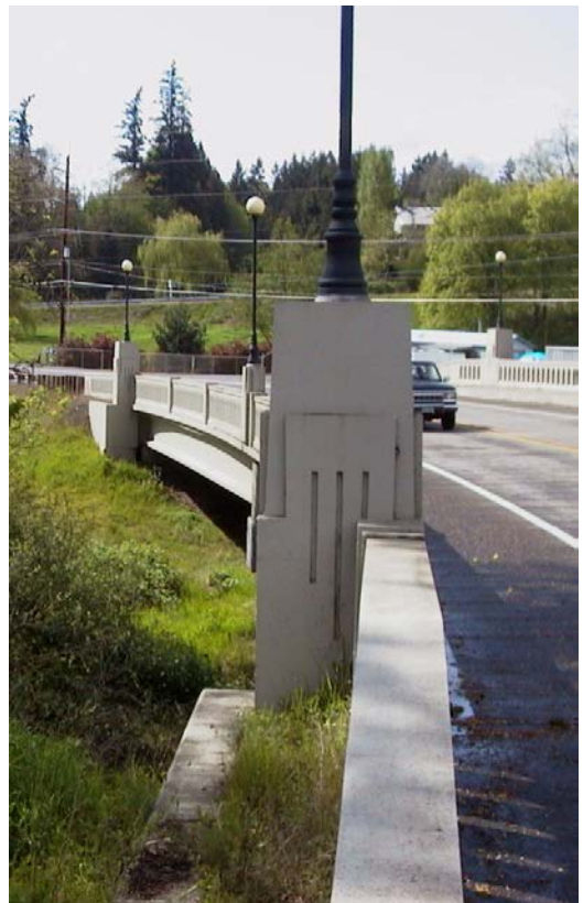
Green retrofits can help intercept rainwater thereby minimizing the negative impacts to streams and other waterways.
