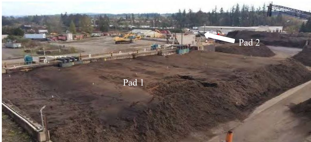
Figure 3: Grimm’s Fuel Company October 2020, both pads are operational.
