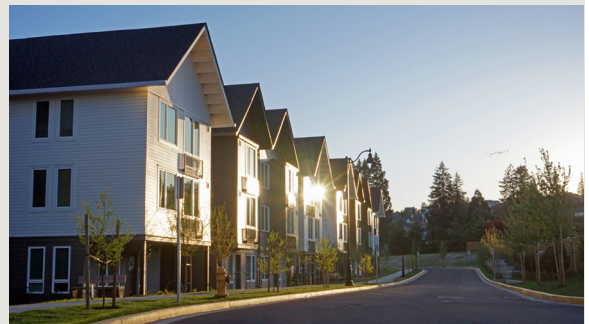
Good Shepherd Village is the first affordable housing to be built in Happy Valley, and the largest affordable housing development in Clackamas County. In November 2023.
