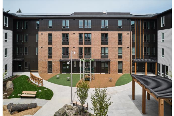
Related Northwest's Crescent Court, example courtyard and landscaping
