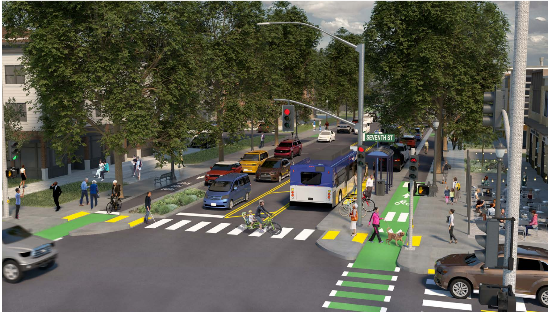
Community street. This rendering illustrates a two-lane minor arterial. The surrounding land use is a neighborhood and this segment of the street functions as a main street. The flex zone includes on-street parking and planted bulb outs.
