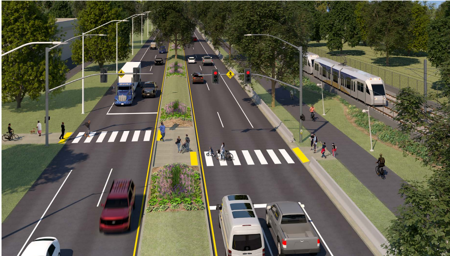
Highway. This rendering illustrates a four-lane throughway that is not grade separated and has some street connections. Land uses are set far back from the highway. The center median increases safety and supports motor vehicle mobility. Parallel light rail and a multiuse path provide transportation options within the corridor. Signalized intersections provide access to the path and light rail stations.
