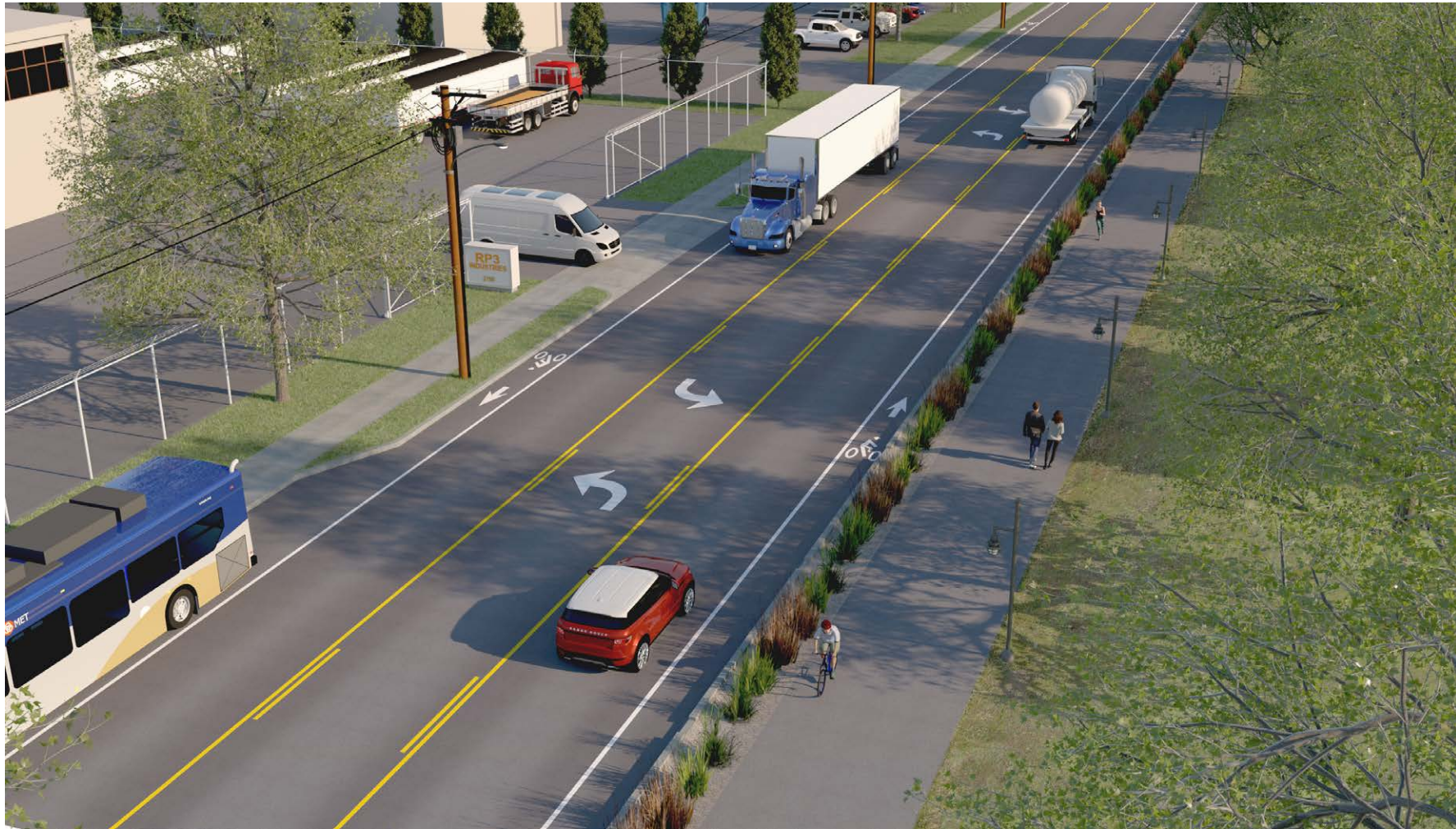
Industrial street. This rendering illustrates a two-lane arterial in an industrial area. Buildings are between one and two stories with large setbacks. A center turn lane and wide driveways accommodate the turning movements of large trucks. A parallel multiuse path increases safety for all users.
