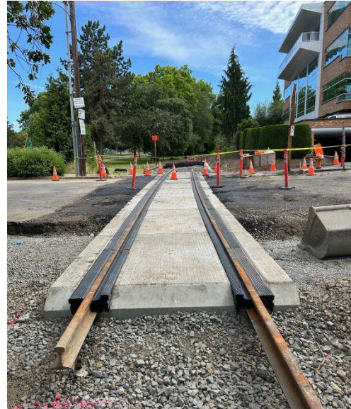
Installed the concrete panel tub at crossing, photo courtesy of TriMet
