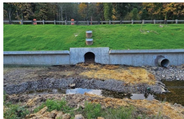
From top: Red-legged frogs need to travel from forests to wetlands and back again in order to breed; the underpass looks a lot like a regular storm drain. Lower photo courtesy of Columbia River Estuary Study Taskforce.
