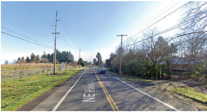
NE Halsey Street - east of NE 192nd Avenue
