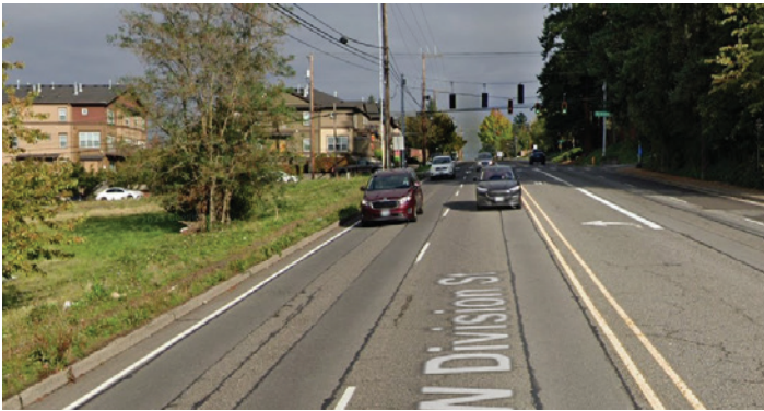
NW Division Street - north side sidewalk gap
