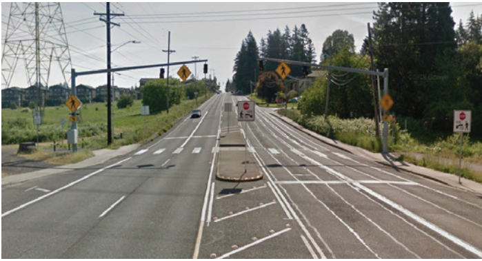
NW Division Street & Gresham-Fairview Trail Crossing
