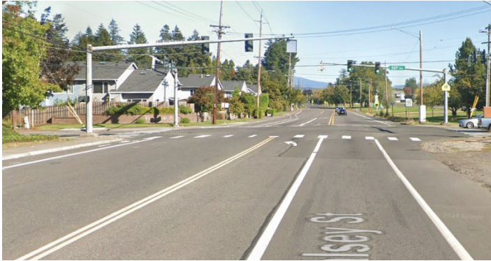
NE Halsey Street & NE 201st Avenue intersection
