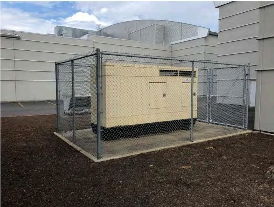
Photograph 22 – Generator with self-contained fuel source near Exhibit Hall E.
