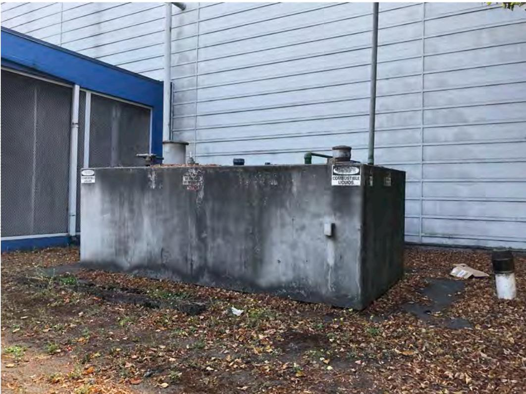
Photograph 20 – 1,000-gallon aboveground diesel tank associated with emergency generator on north side of Exhibit Hall B.
