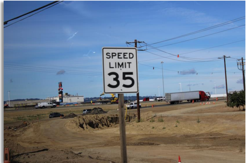
Construction at the Aurora-Donald Interchange
